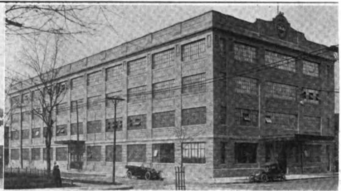
The Stutz Motor Car Co., Indianapolis, Ind., has occupied an entirely new factory building which increases its floor area 60,000 square feet at a cost of $100,000
